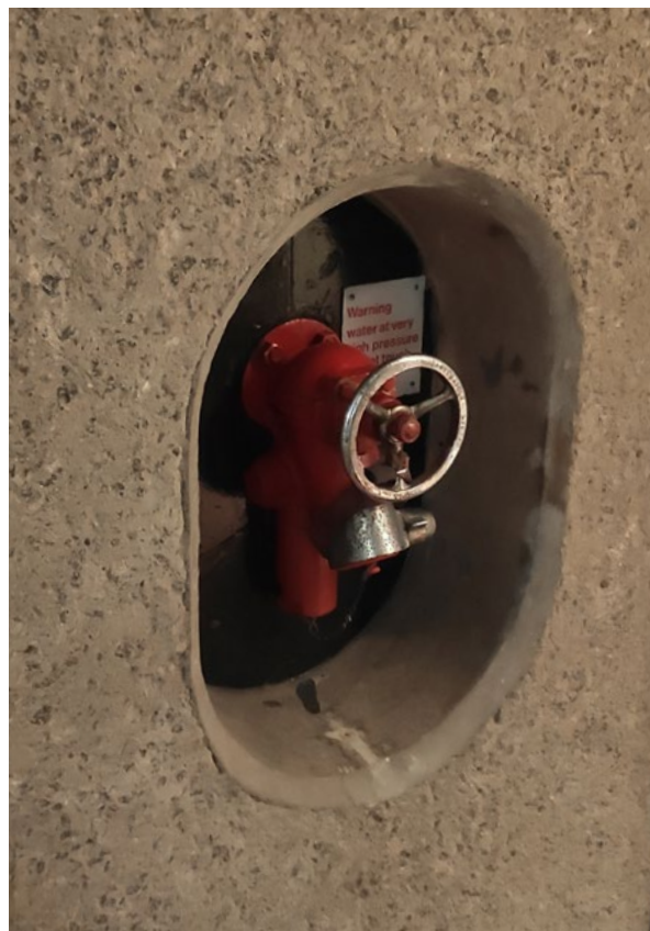
Recessed wet riser in concrete wall
